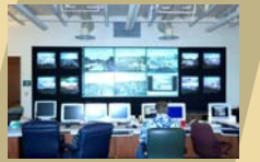
Traffic Management Center
